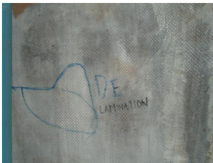
Figure 9b. Delamination and worn out
