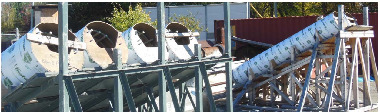
Figure 6. The B.P specimens on the formwork.
