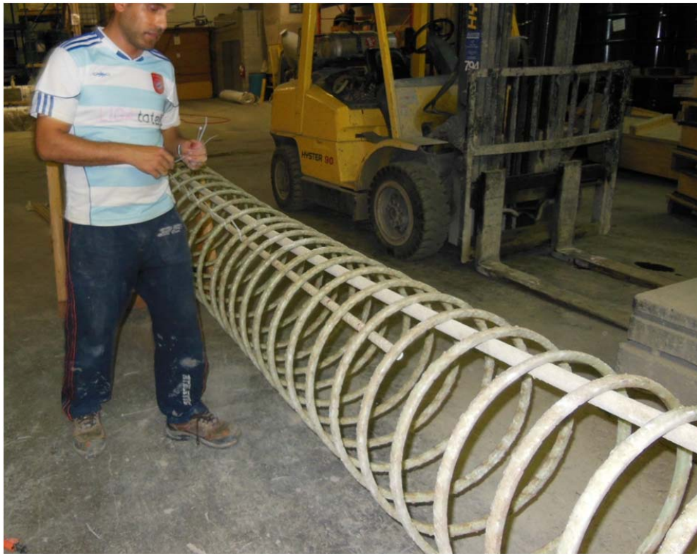
Figure 3. Preparing of B.P GFRP cages.
