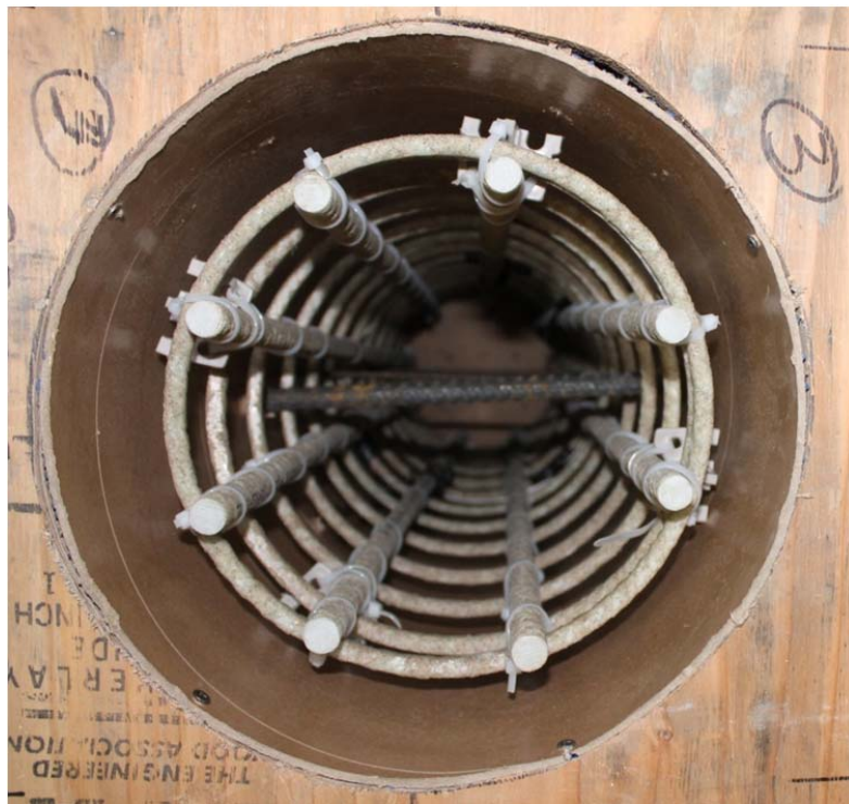
Figure 13. Overview for cages inside formwork
