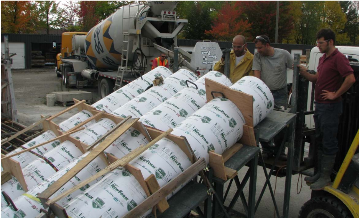
Figure 7. Casting of circular beams.
