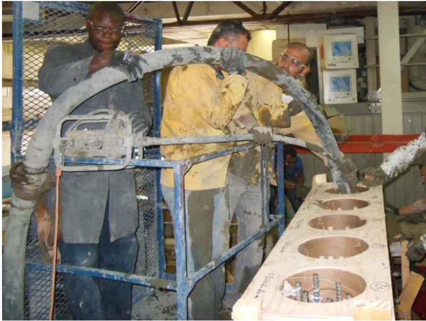
Figure 14. Casting of columns
