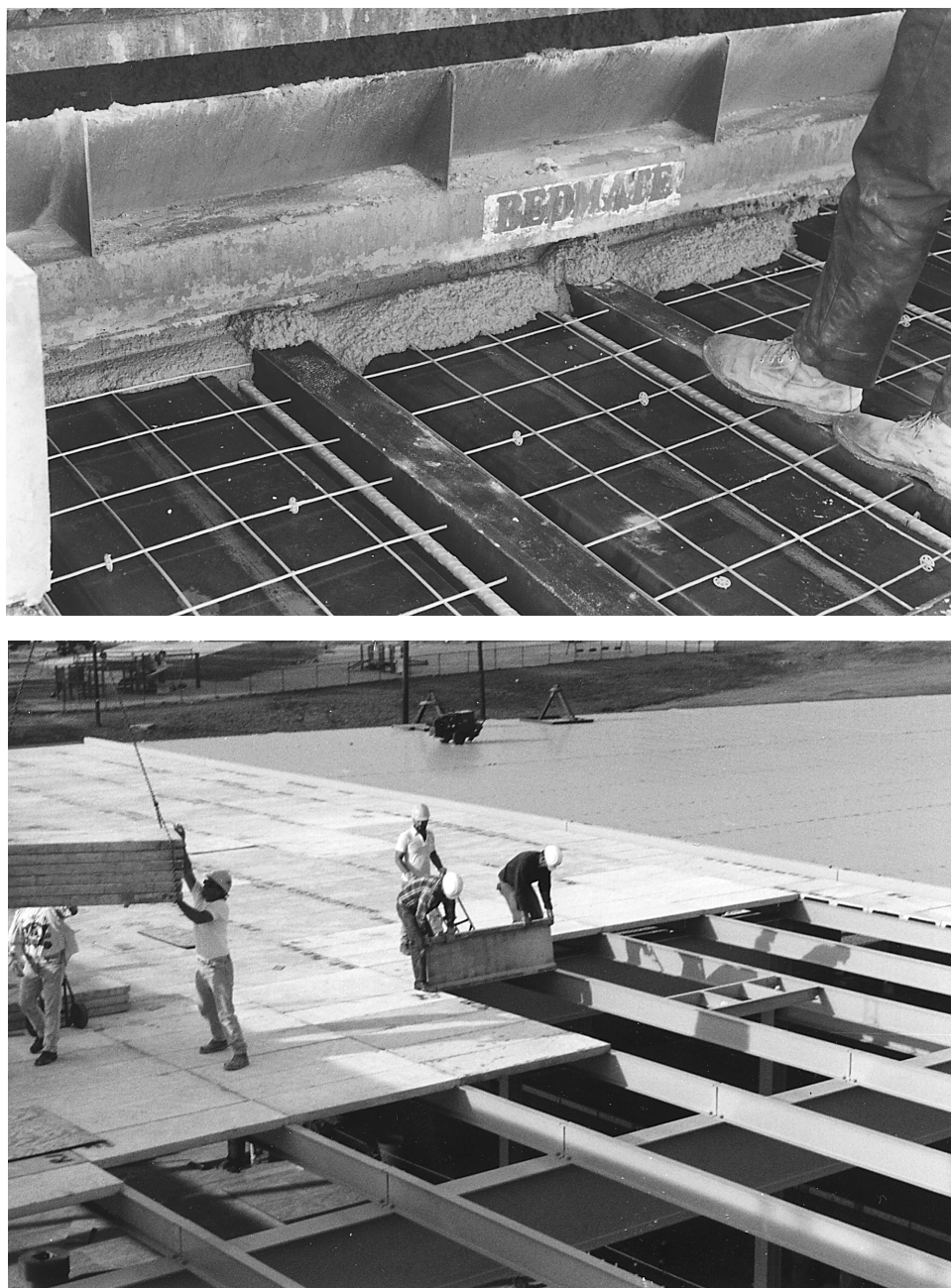
Fig. 8.4—Construction and placement of precast channel slabs, Atlanta, Georgia
