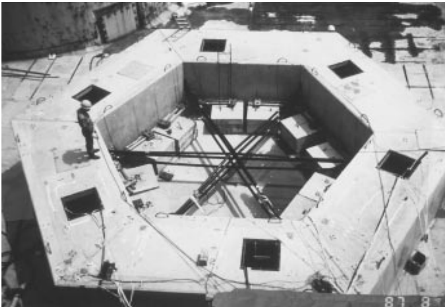
Fig. 8.13—Hexagon marine structure, Kanagawa, Japan
