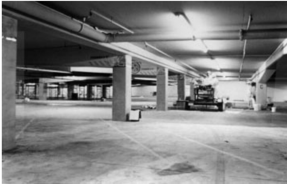
Fig. 8.15—Columns strengthened with GFRP, Reno, Nevada
