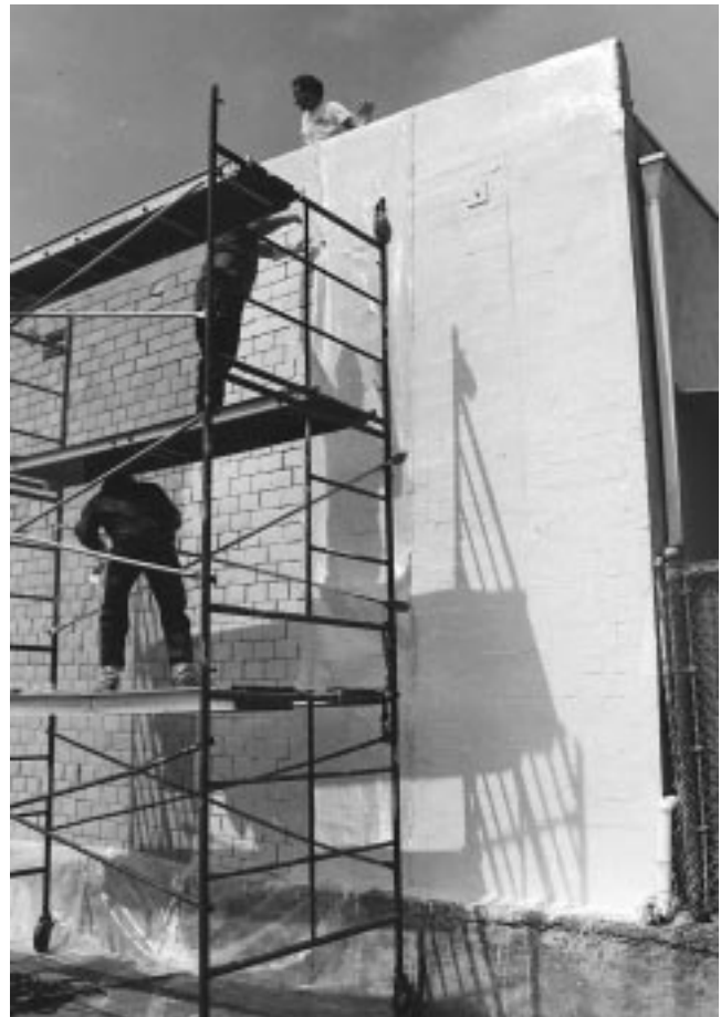
Fig. 8.16—Seismic retrofitting of unreinforced masonry wall in California
