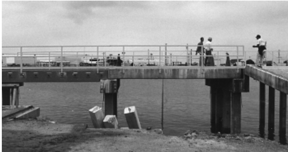
Fig. 8.8—Waterfront structure, Port Hueneme, California
