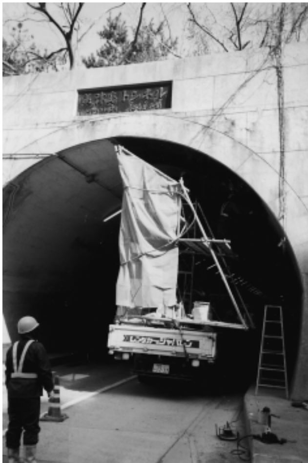
Fig. 8.20—Application of Forca Tow Sheet inside tunnel, Japan
