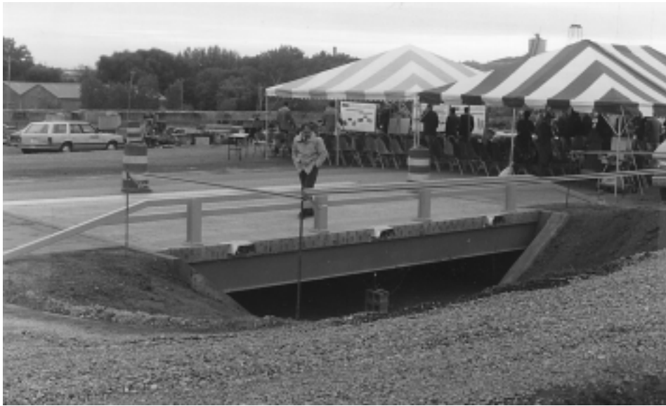
Fig. 8.7—Composite prestressed bridge at Rapid City, South Dakota
