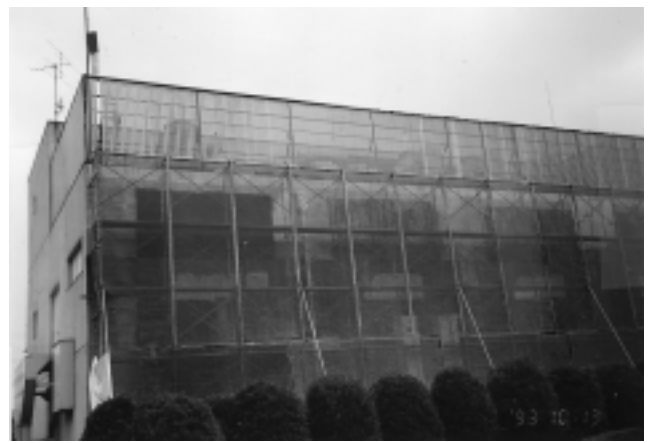
Fig. 8.21—Overview of building wrapped with Forca Tow Sheet, Japan
