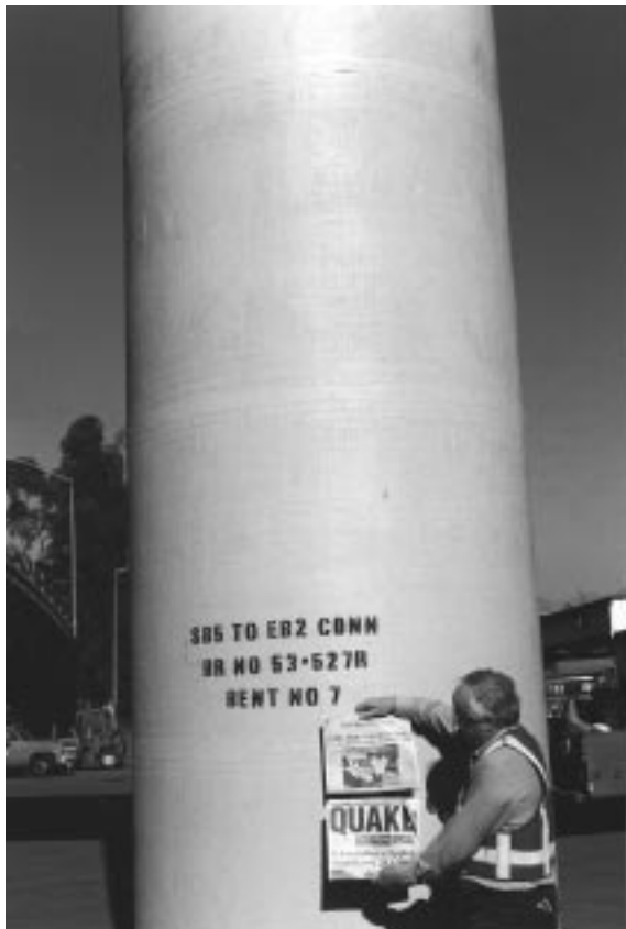
Fig. 8.14—Bridge column wrapped with GFRP, California
