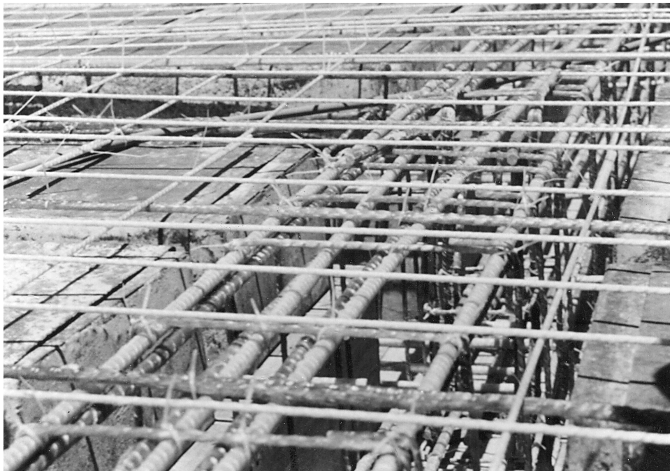
Fig. 8.3—Hospital building, San Antonio, Texas
