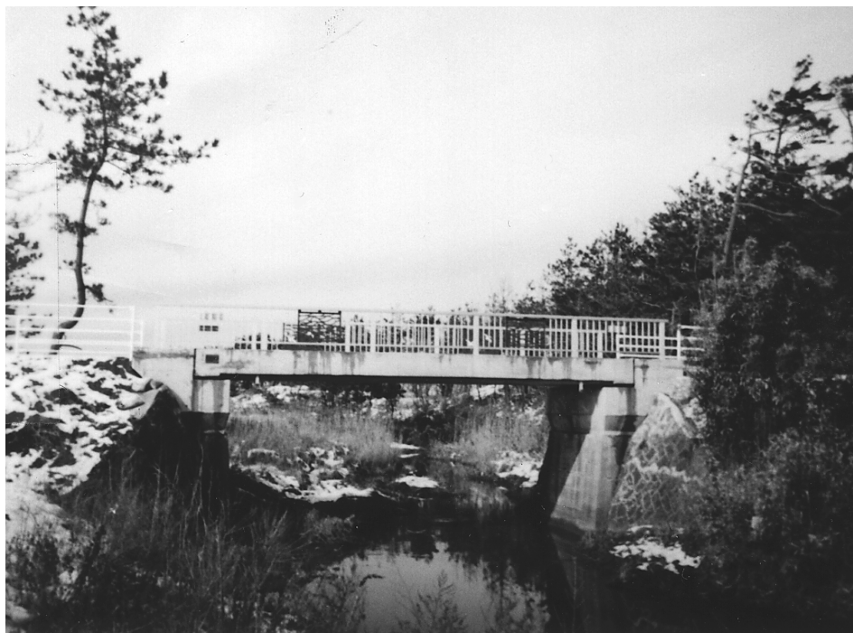
Fig. 8.11—Shinmiya Bridge, Japan
