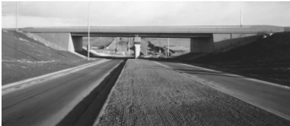
Fig. 8.6—Bridge at Calgary, Canada
