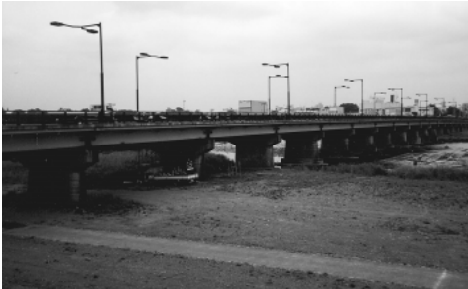
Fig. 8.19—Overview of bridge rehabilitation with Forca Tow Sheet, Japan
